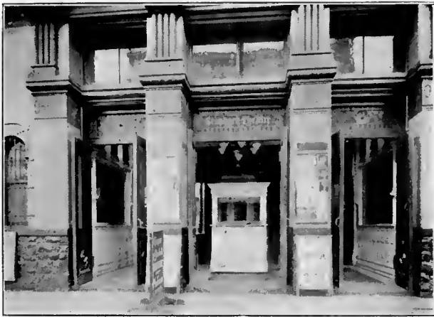
LOBBY ENTRANCE & TICKET SELLER'S BOOTH
